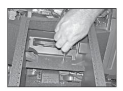
Place the two screws back into lower center holes.(but do not tighten down)
