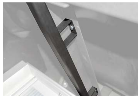
Install Secure Grid Support Tubes using provide (2) 7/16 hex bolts. REPEAT FOR OTHER SIDE.
