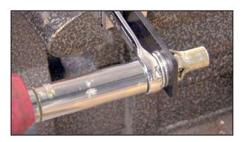
5. Apply pressure on the flange nut, pressing AVK Fastener into hole.
