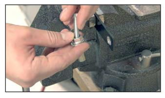
2. Place  $5/16-18 \times 1.5$ " long bolt through the 3/8" flange nut and hand thread bolt into the AVK Fastener.
